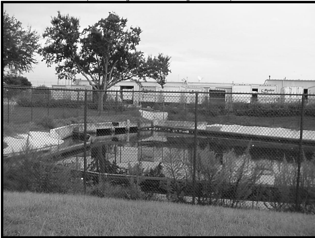
Figure 4-66. Settling Pond for Alum Treatment System
