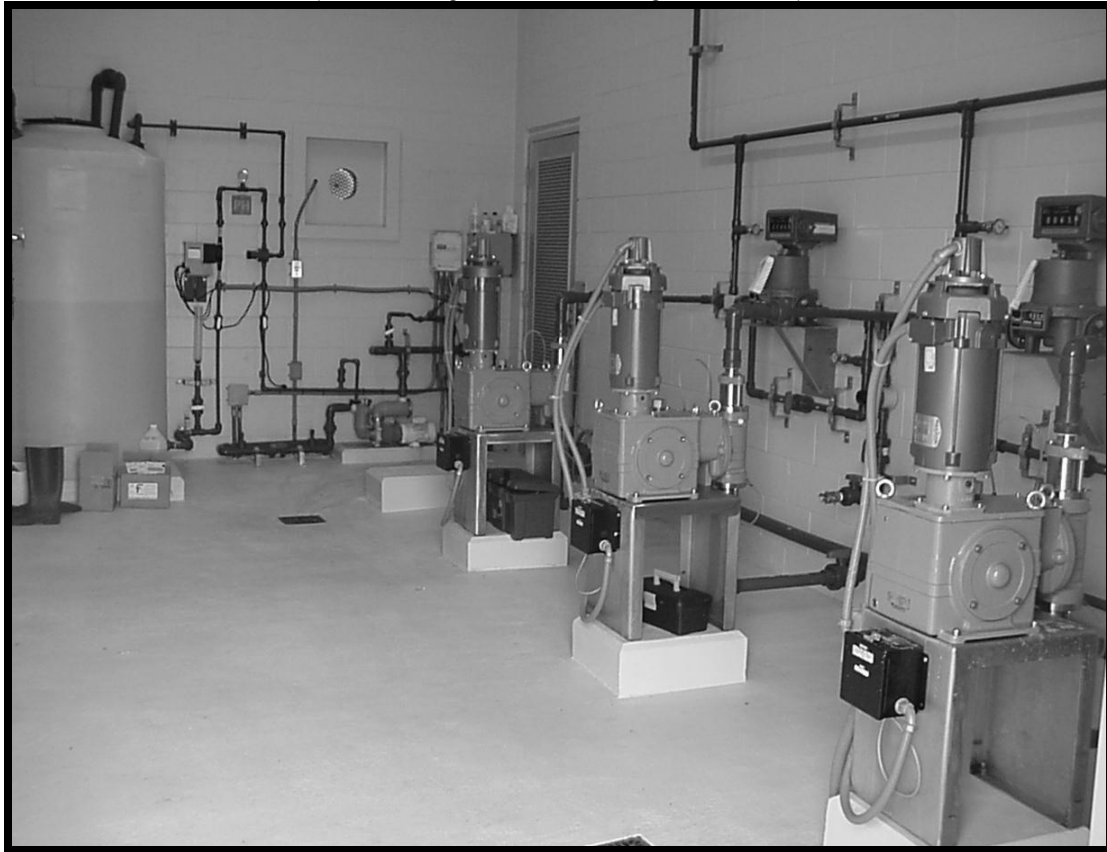
Figure 4-67. Dosing/Injection Components of an Alum Treatment System
